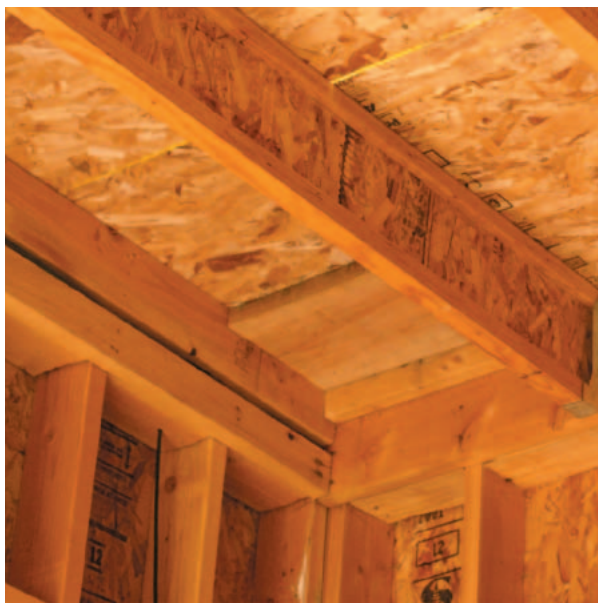
Figure 17-36 Ceiling Framing
