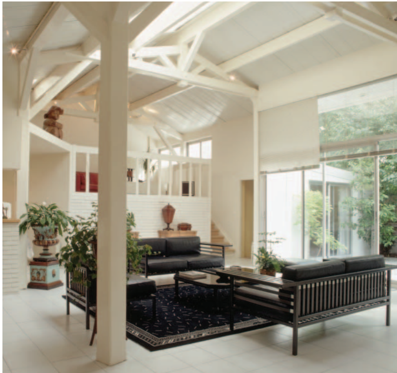
Figure 17-47 Roof Trusses An Open Floorplan Because these trusses would be exposed to the living space, the truss builder took extra care to make them visually appealing.
