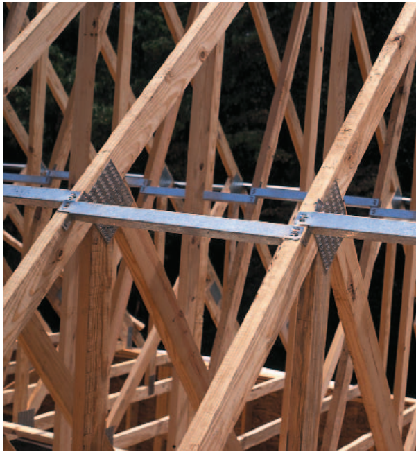
Figure 17-50 Truss Bracing Double Duty Prefabricated metal spacers help to brace trusses and ensure exact spacing.
