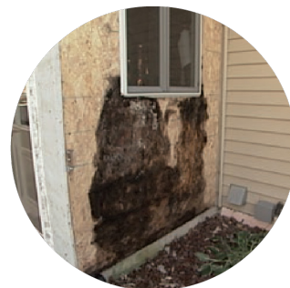
House rot from improper moisture management
